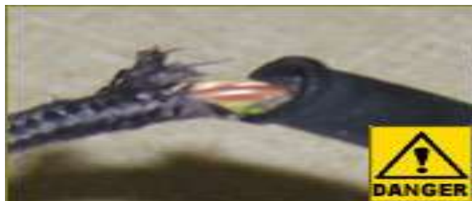
Electrical equipment with damage cord
